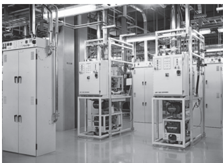
GRC technology has been used to abate the exhaust gas streams on a wide range of semiconductor applications. (Photograph courtesy of TI, Dallas, USA.)
